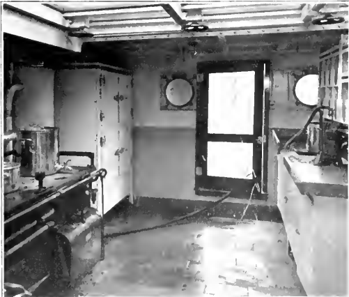
The galley of the Columbine featuring the Ingle range and Frigidaire cabinet.
